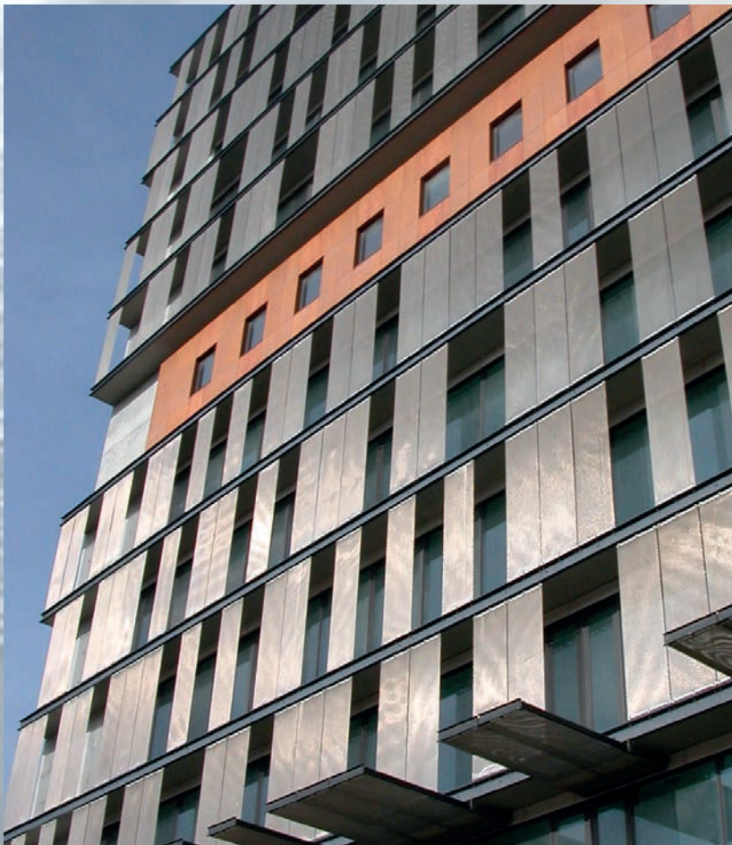
Transparent architectural mesh elements effectively combine sun protection with superb design possibilities.
