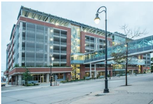
2. Carlisle Bridge View.jpg
